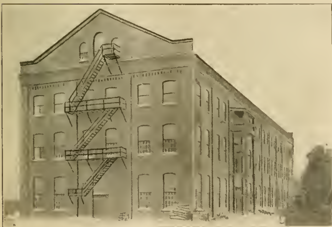
CARPENTER-SHOP BUILDING, SHOWING OUTSIDE STEEL CONSTRUCTION FOR ELEVATOR SERVING THE PATTERN LOFTS.
